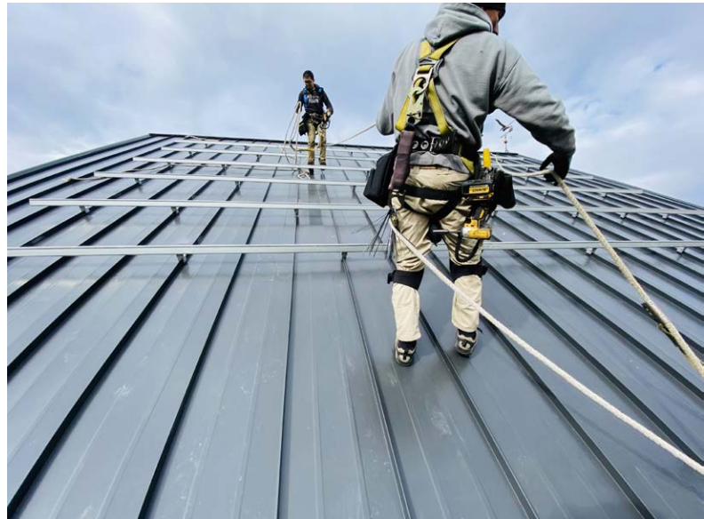
Solar installers on roof. Photo credit: A&R Solar
