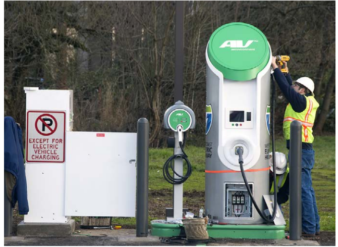
Worker assembling charging station. Photo credit: Oregon Department of Transportation
