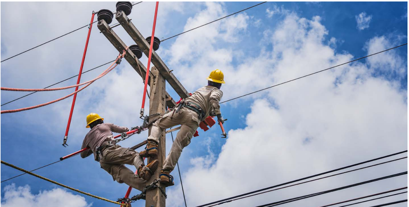
Electrical lineworkers preparing to replace damaged high-voltage insulator. Photo credit: 3asy60lf
