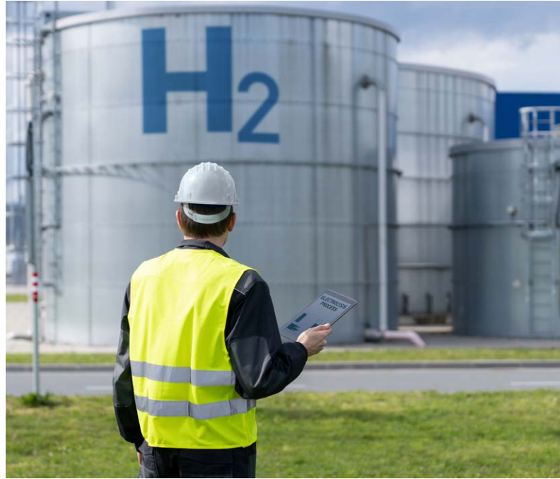
Engineer in front of hydrogen facility. Photo credit: scharfsinn86
