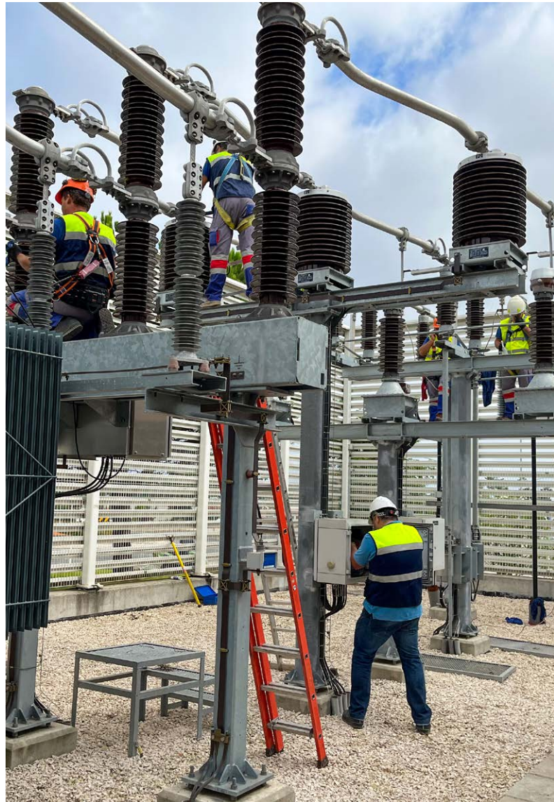
Maintenance in a high-voltage electrical substation. Photo credit: Paulo Esteves
