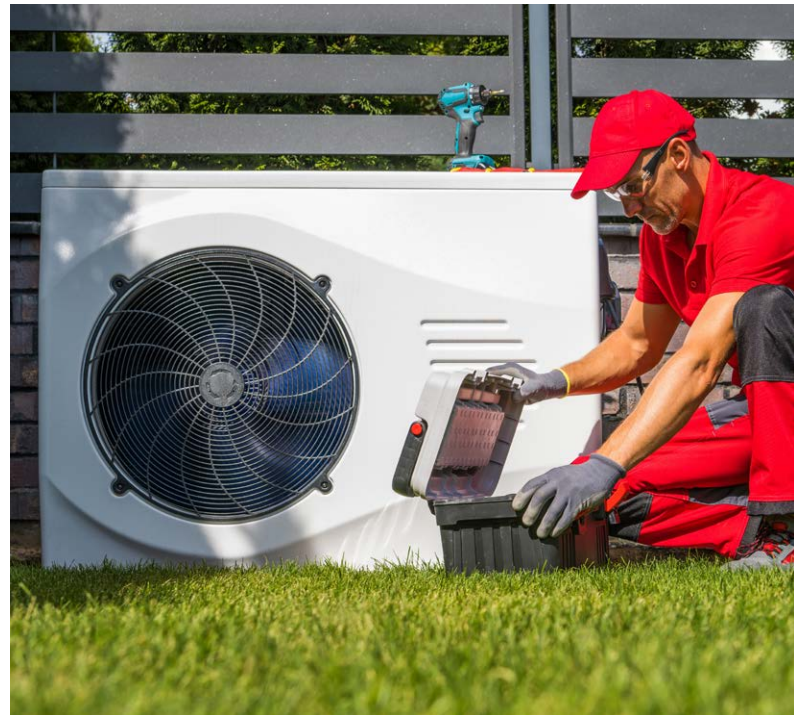
Heat pump technician installing new device. Photo credit: Tomasz Zajda
