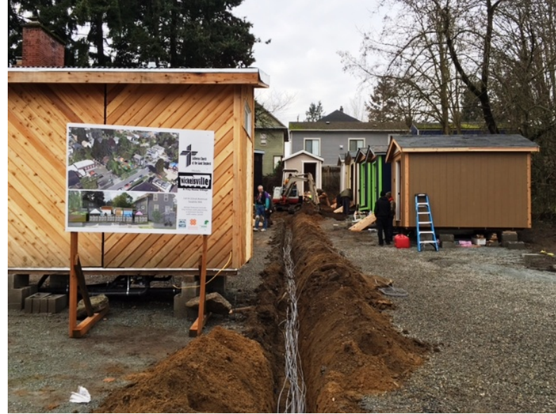
Electrical Cable Trench
