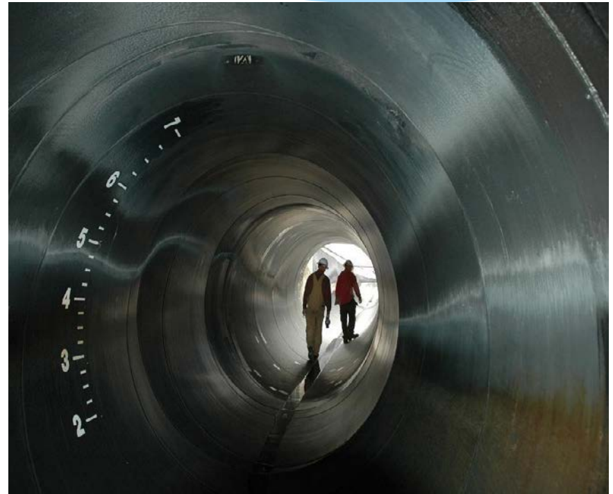
Maintenance employees walk through the junction Photo courtesy of Chelan County PUD
