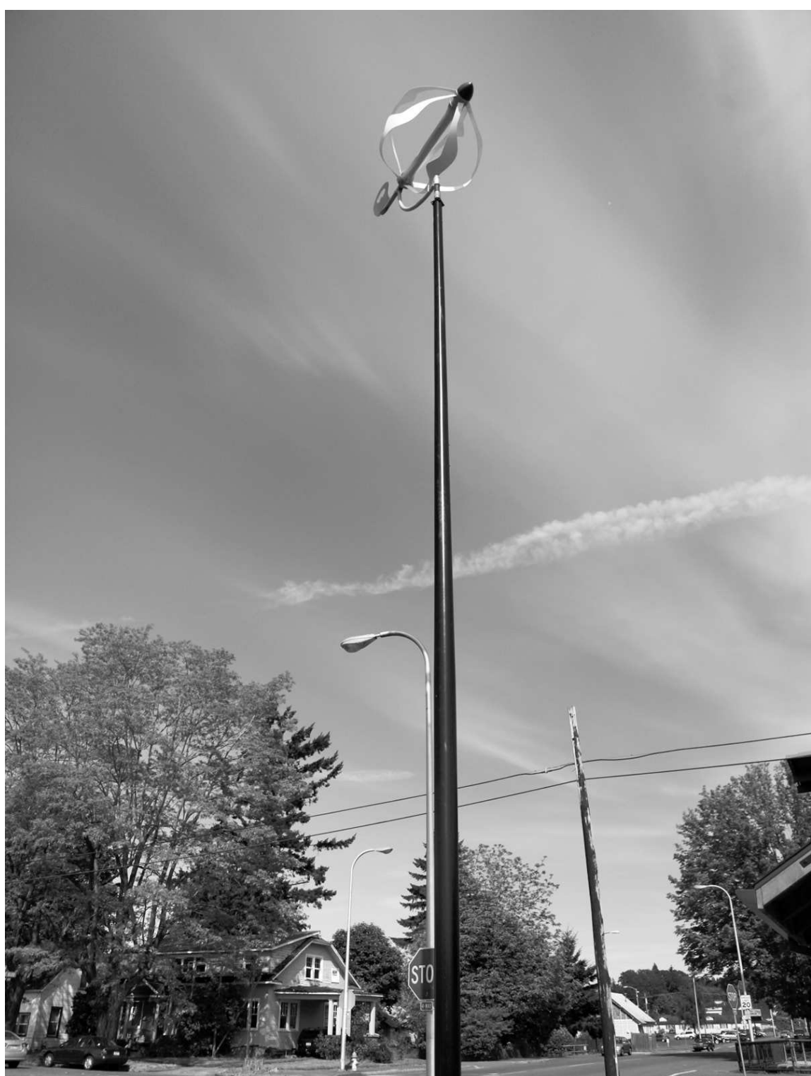
A wind turbine now stands at the corner of Washington Avenue and Centralia College Boulevard that will feed electricity into the city's power grid any time the wind is blowing faster than 6.7 miles per hour.
